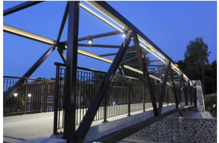
50 watt LEDs. The LED engine provides 4000 lumens, with a color temperature of 4100 kelvin.
