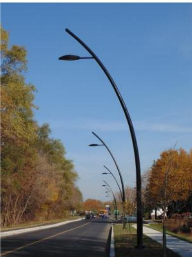
The contemporary Adelo Series was chosen and installed on a curved aluminum pole recalling the davit arm traditional look.
